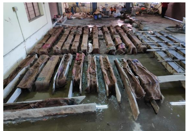
FIG 6 CURING OF BEAMS
