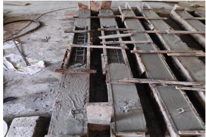
FIG 5 CASTING OF BEAMS
